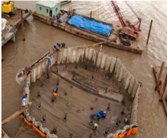
Figure 2.12 Cover around foundation with canvas
