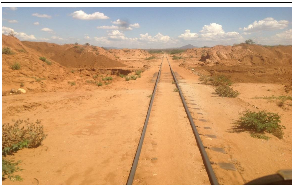
Figure 4-4 Heaps of Sand/Soil recovered from a bridge in the existing MGR at Gulwe (Mpwapwa) as a result erosion upstream
