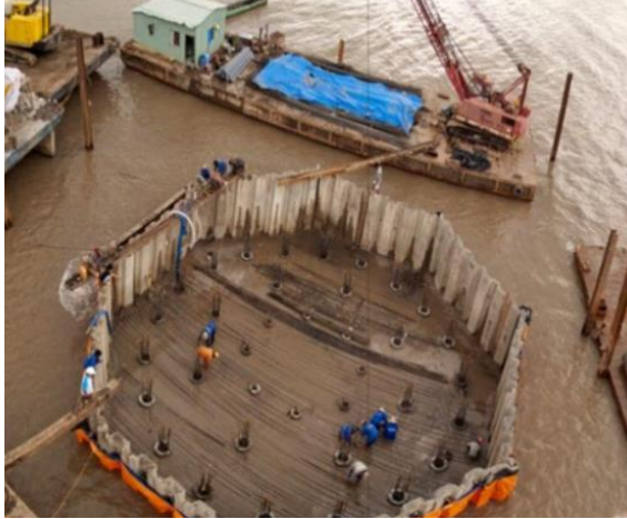
Figure 2.12 Cover around foundation with canvas
