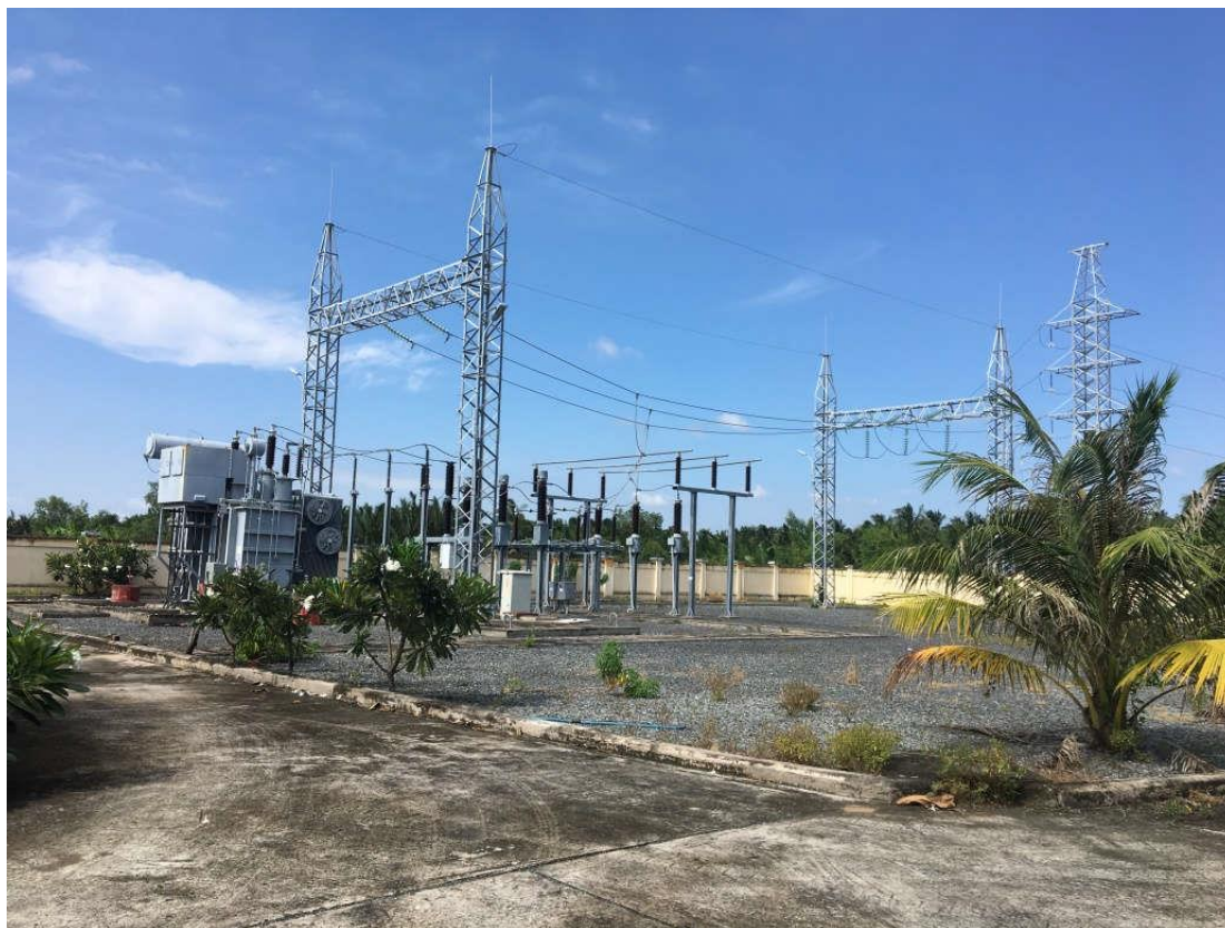
Figure 2.7 The connection area of 110kV Binh Thanh Substation
