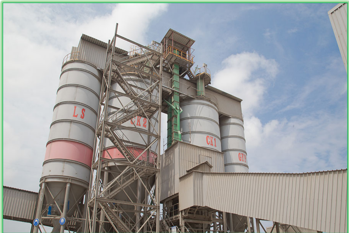
Figure 3-8: Existing raw material silos
